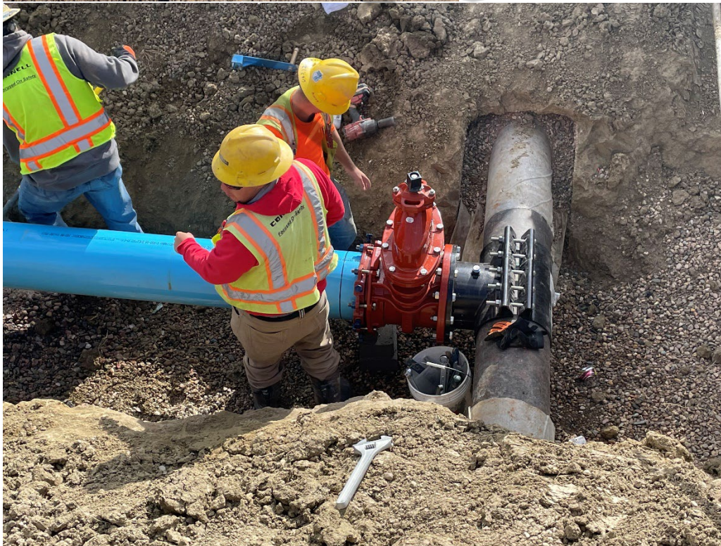
Left: Tapping saddle and valve on existing discharge pipe from APS. Below: First stick of pipe(12") installed into tapping valve.
