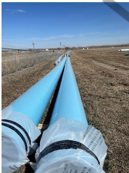
Left: Suction line (left) and discharge line (right) - each ~900 ft long. Right: The two fusing machines set up near the middle of the project.
