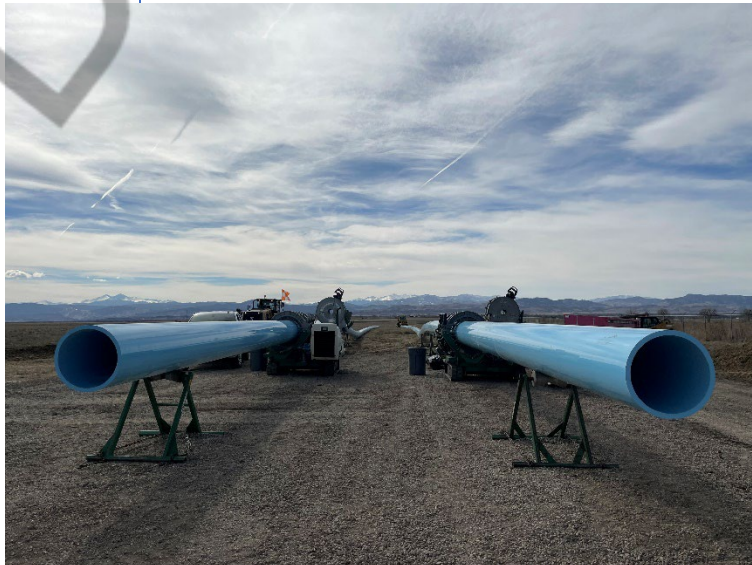
Left: Suction line (left) and discharge line (right) - each ~900 ft long. Right: The two fusing machines set up near the middle of the project.
