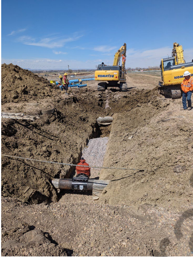
Left: Tapping saddle and valve on existing discharge pipe from APS. Below: First stick of pipe(12") installed into tapping valve.
