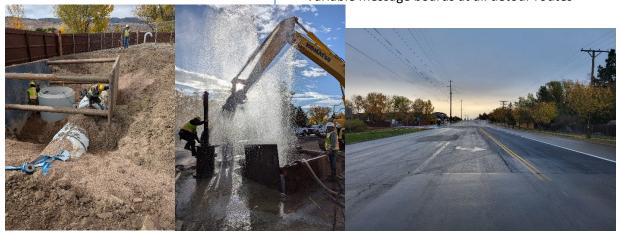
Left: 42" Butterfly Valve Vault Center: Line stop removal Right: Final pavement and striping
