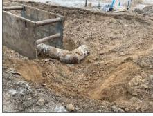
Left: Backfill of 30" waterline in cold weather
