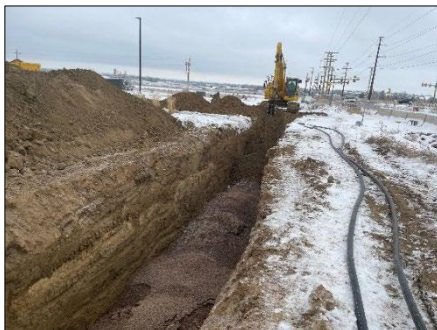
Left: Backfill of 30” waterline in cold weather
