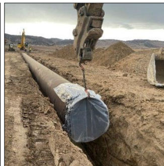
Center: Installation of steel casing for future Transfer Station access roads
