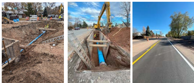
Left: 8" service tie-over into Capital Drive
