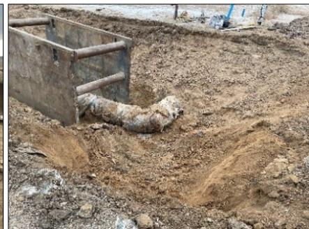
Right: Existing 24” 90 degree bend and tie in location for the 30” feeder pipe line to the existing 4 MG Tank
