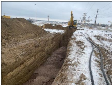
Left: Backfill of 30” waterline in cold weather
