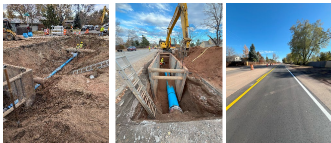
Left: 8" service tie-over into Capital Drive
