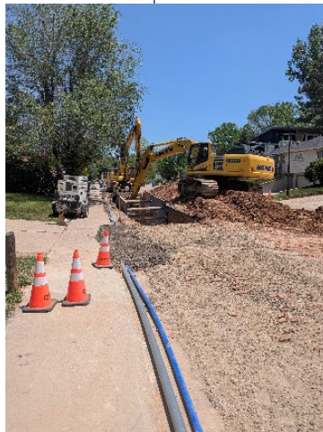
Center: Installation of waterline with dewatering piping
