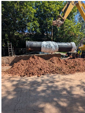
Left: Installation of 42" DI Waterline
