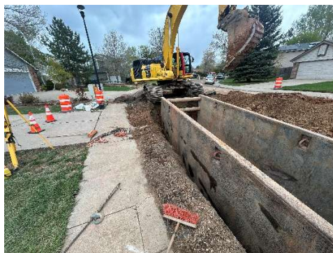
Left: Trench excavation along Virginia Dale
