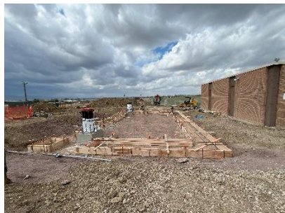
Left: Forms for concrete footer
