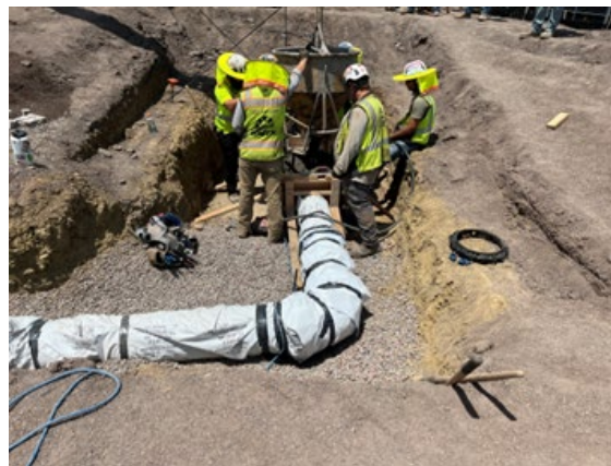
Right: Pouring concrete for site piping encasement
