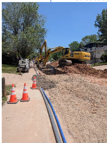
Center: Installation of waterline with dewatering piping
