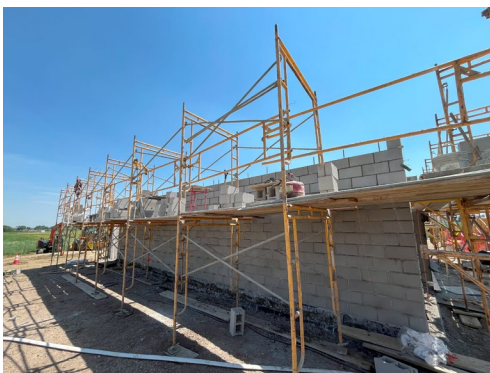
Left: West CMU walls being constructed
