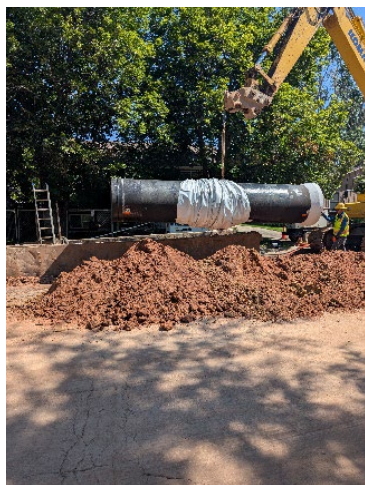
Left: Installation of 42" DI Waterline
