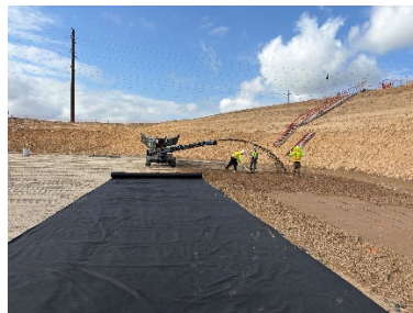
Center: Installation of Geotech fabric under the tank base
