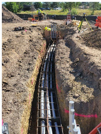
Left: Installation of site electrical duct bank
