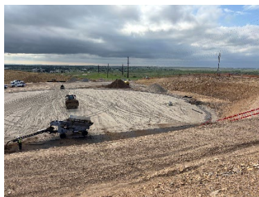
Left: Installation of CDOT Class 6 base
