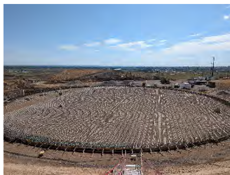
Left: Tank floor rebar and PT duct.
