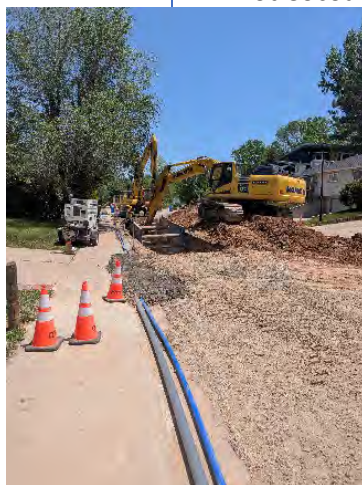
Center: Installation of waterline with dewatering piping
