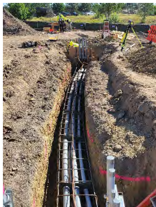
Left: Installation of site electrical duct bank
