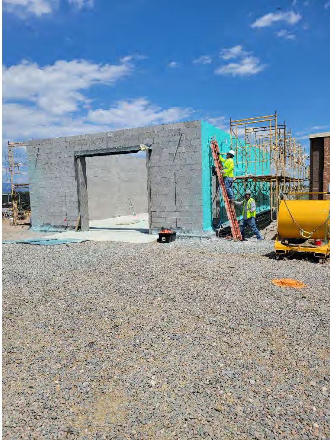
Above: Placing vapor barrier on the CMU walls
