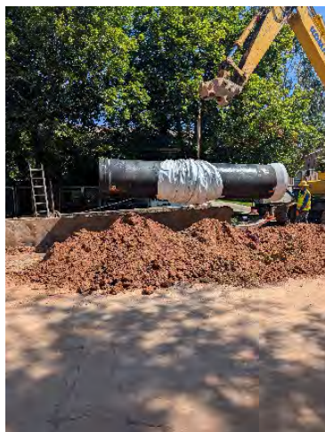
Left: Installation of 42" DI Waterline
