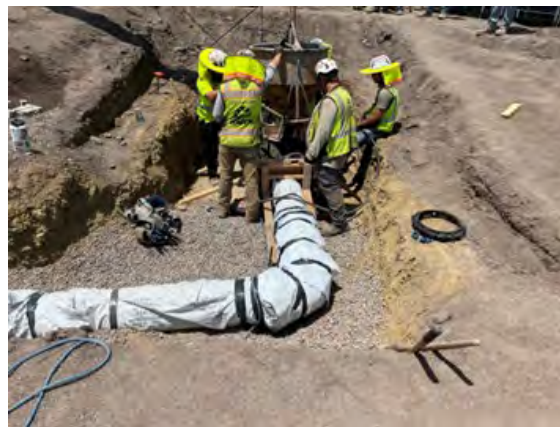
Right: Pouring concrete for site piping encasement
