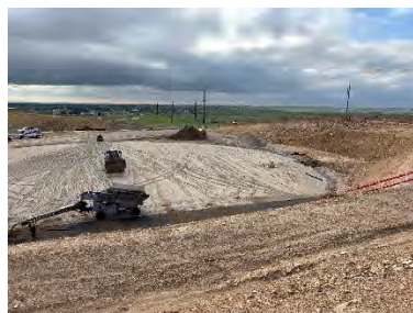
Left: Installation of CDOT Class 6 base
