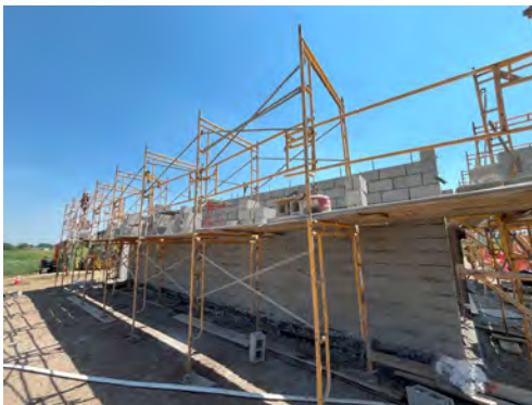
Left: West CMU walls being constructed
