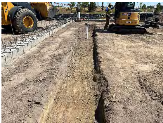
Left: Preparing for installation of the interior trench drain Right: Backfilling concrete foundation
