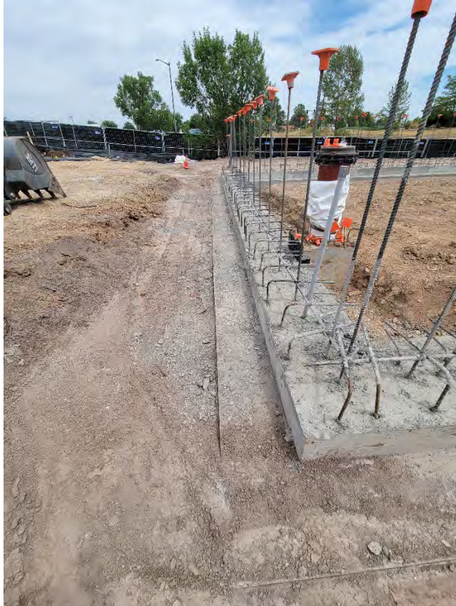
Above: Building concrete foundation placed
