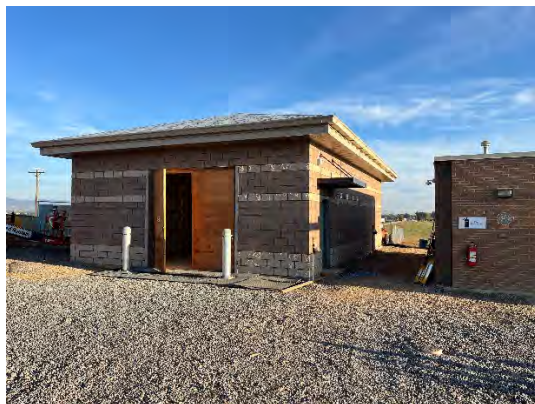
Left: Exterior soffit, fascia, and gutter installation
