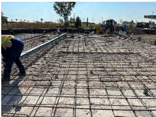
Left: Placement of reinforcement for the buildings concrete slab on grade
