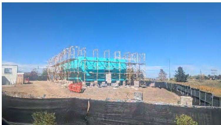
Left: Placement of damp proofing on CMU block
