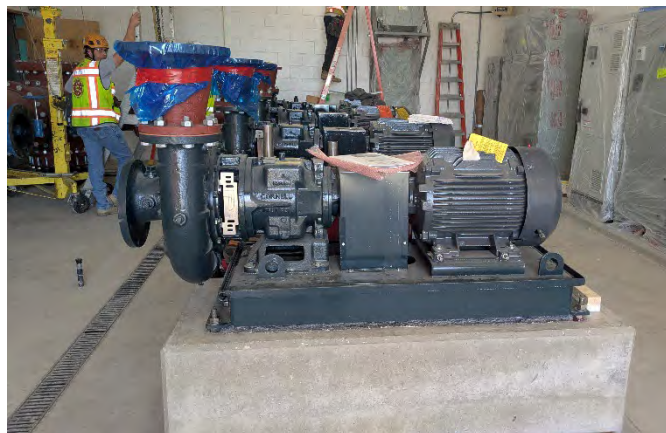
Above: Installation of pumps
