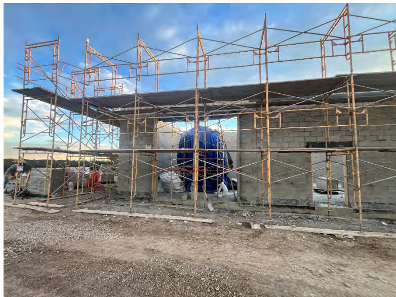
Above: Installation CMU Structural block
