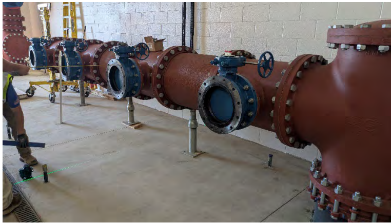
Above: Interior process piping being installed
