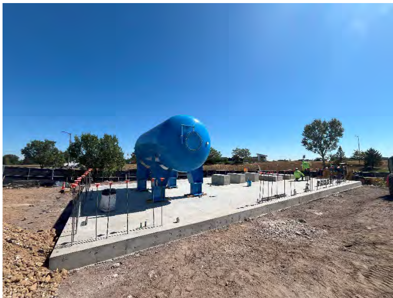
Above: Installation of the surge tank
