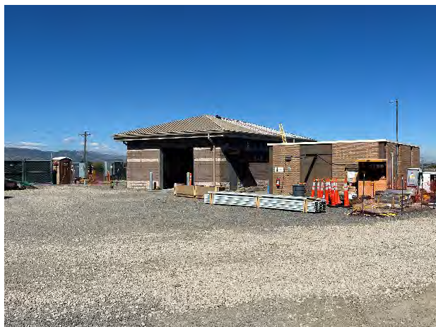
Left: Metal roof panels being installed
