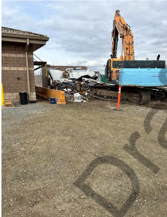
Above: Demo of the existing pump station
