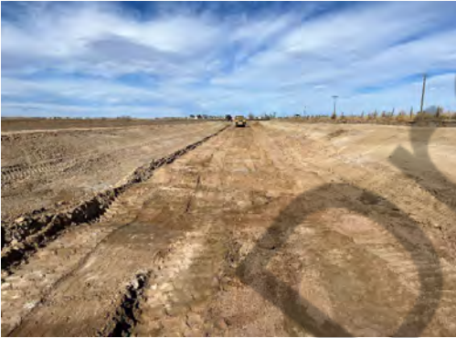
Above: Recharge Cell #1 being cut to grade.
