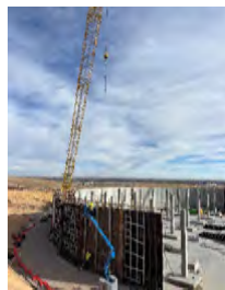
Left: Placement of concrete form work in preparation for the 7 th wall pour Center: Crane flying in rebar in preparation for the 8 th wall pour Right: Concrete column base and column form work
