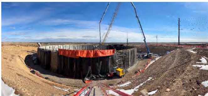
Left: Setting up the last form for the last 3 wall pours and pouring 9 th wall section Right: Setting column reinforcement using the larger crane
