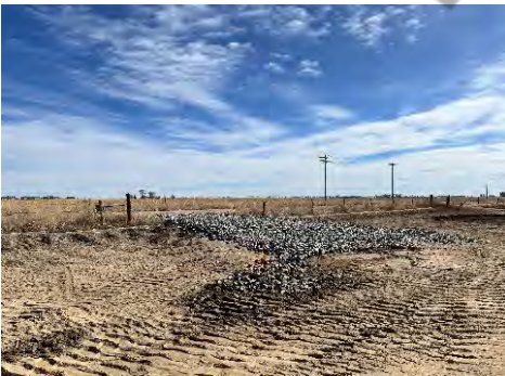
Left: Entry to the construction site established.
