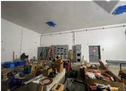
Left: Installation of electrical equipment
