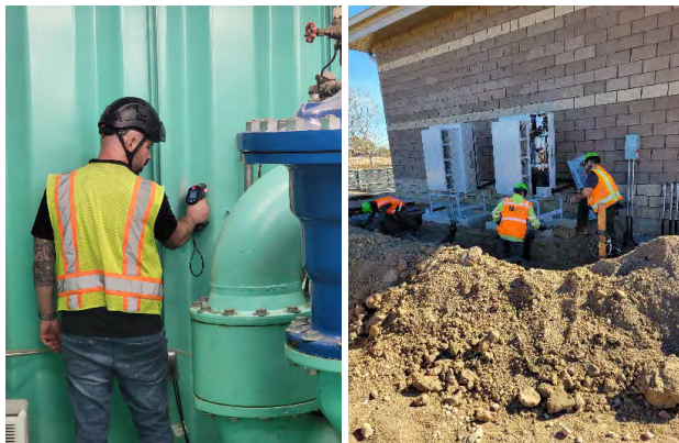
Left: Testing of existing pump station for lead paint.
