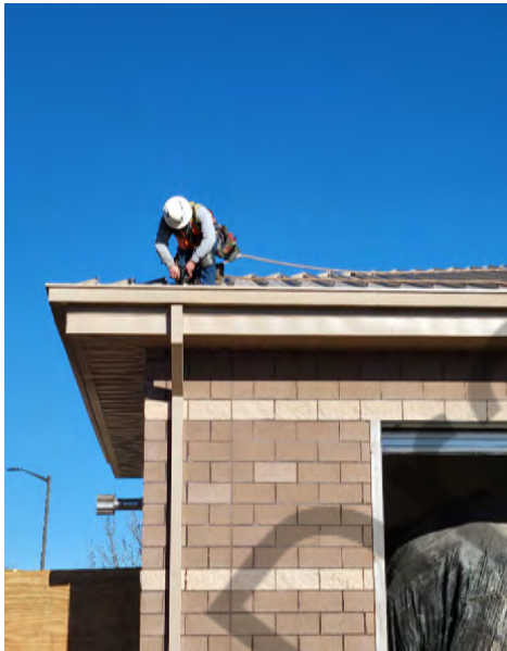
Above: Roofing being installed
