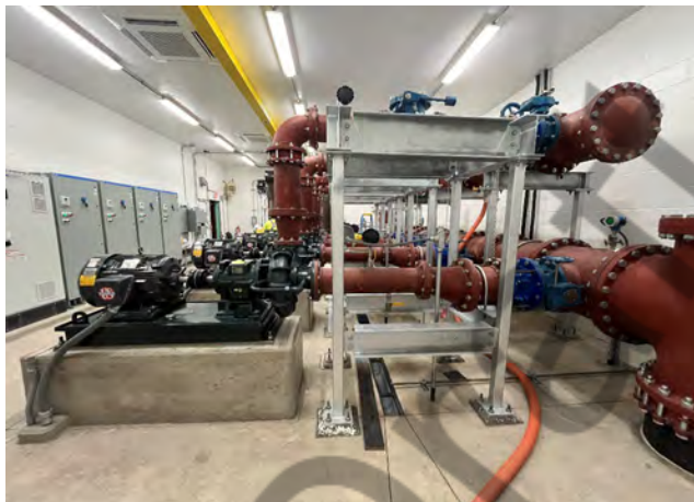
Above: Installation of pipe supports complete
