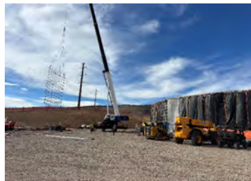
Left: Placement of concrete form work in preparation for the 7 th wall pour Center: Crane flying in rebar in preparation for the 8 th wall pour Right: Concrete column base and column form work
