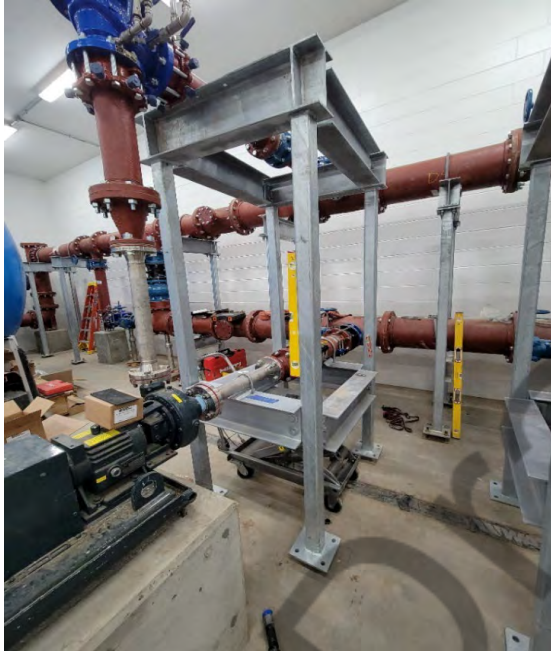
Above: Interior process piping and pipe supports being installed.
