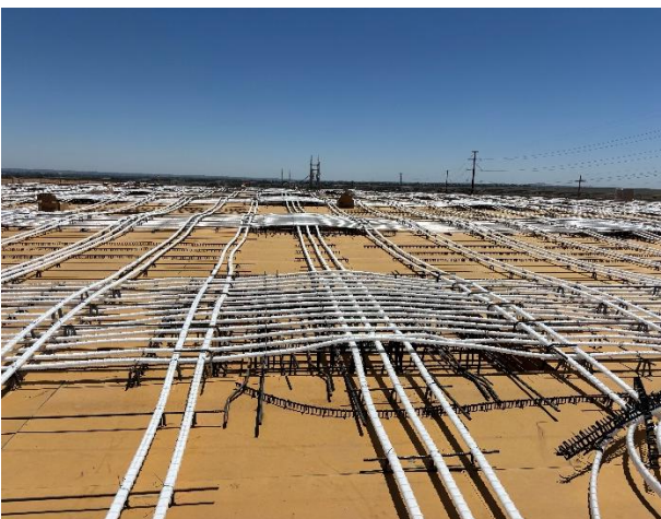
Right: Roof slab reinforcing and tensioning cable conduits Left: Overall tank structure
