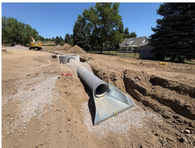
Above: Started onsite stormwater system.
